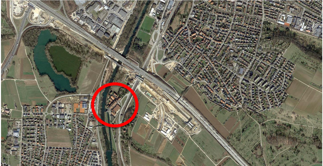
Aerial view of detailing area 2, in red circle the territory of the old cotton mill
