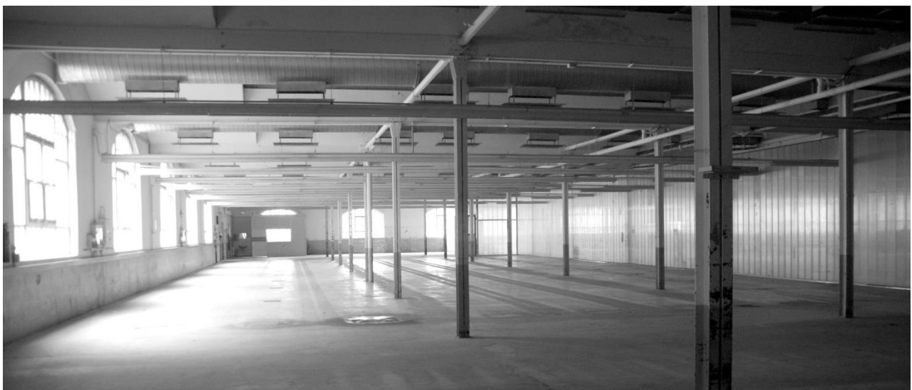
The manufacturing areas of the cotton mill are under heritage protection
