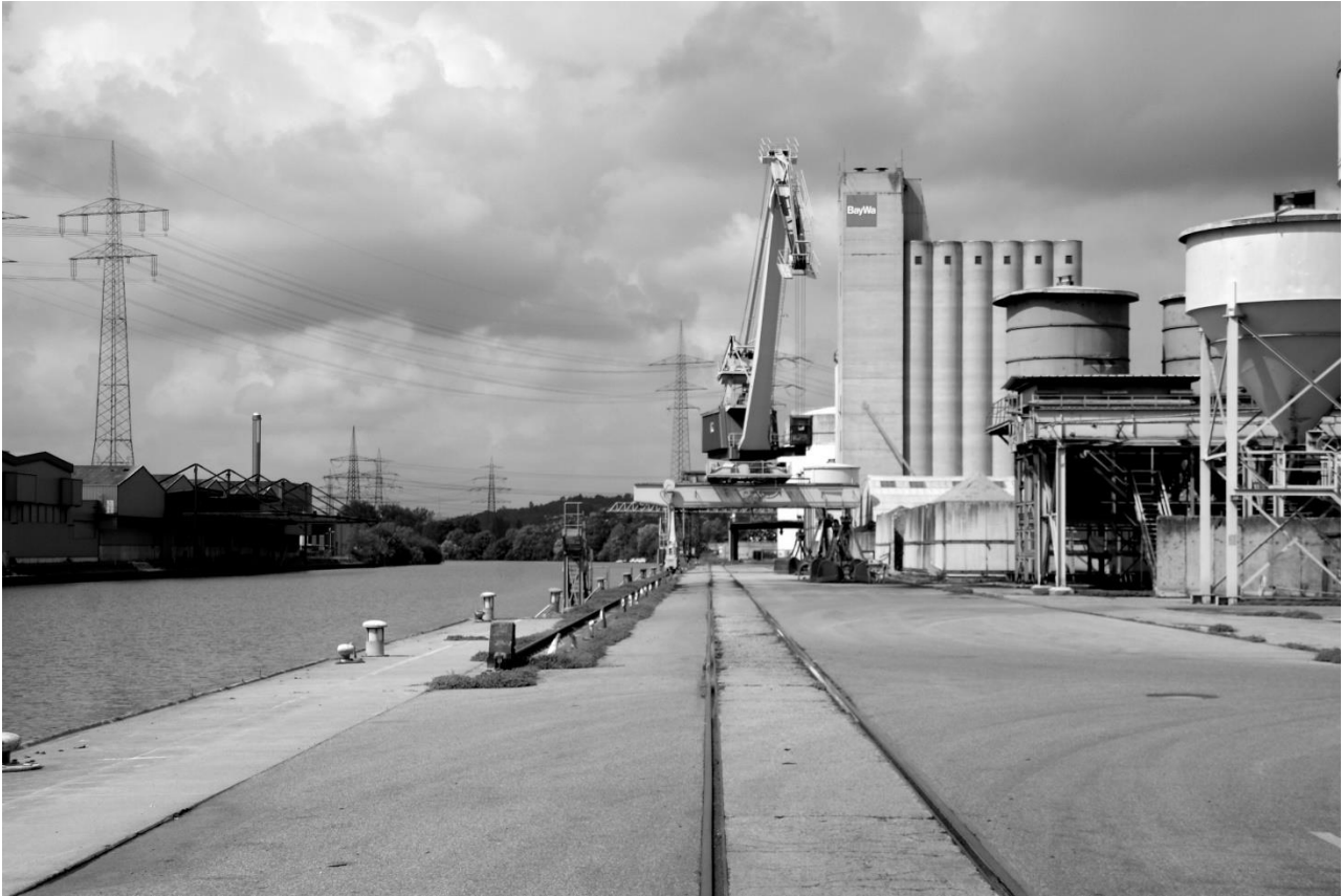
Inside Plochingen harbour, view downstream on the harbour facilities
