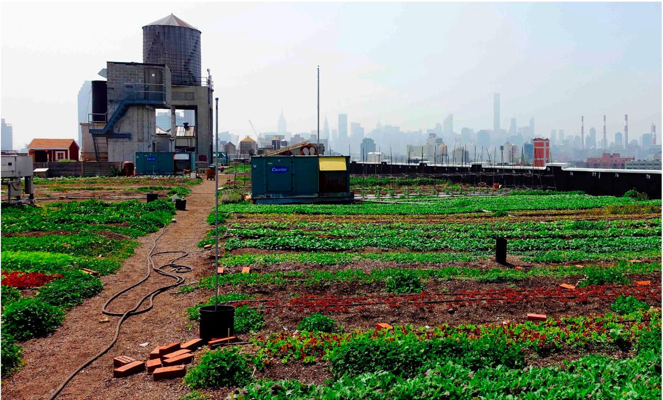
**Figure 10.** View of Brooklyn Grange, New York City. This project demonstrates a green infrastructure approach, reducing stormwater and urban heat island effect. Image from authors.
