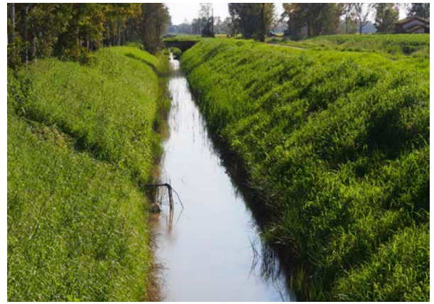
Fig. 35_ Drainage ditches are a common feature
