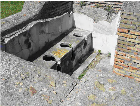
Fig. 1_ marble plates cover the brick masonry
