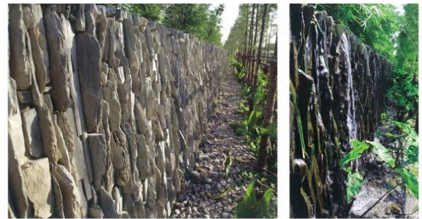
Fig. 47_ Cascade aerates and cleanses river water
