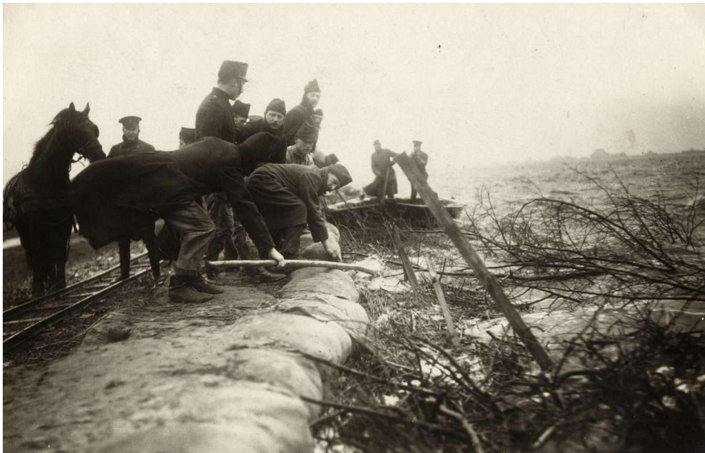
Kees Hofker (1886-1936) - [SFA022813700, Het Leven, Spaarnestad Photo] The flood of 1916. Soldiers and civilians are deployed to establish emergency sea defences. Sacs filled with clay and sand are placed and covered with soil. Anna Paulownapolder, Netherlands, 1916.
